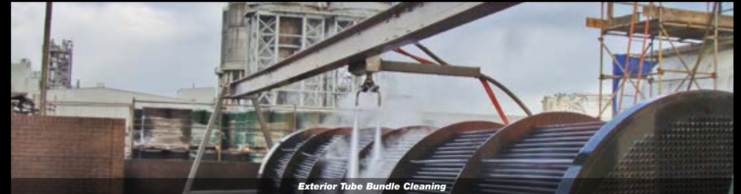
Exterior Tube Bundle Cleaning
