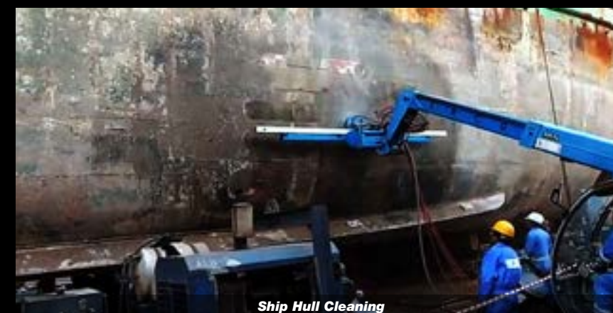
Ship Hull Cleaning
